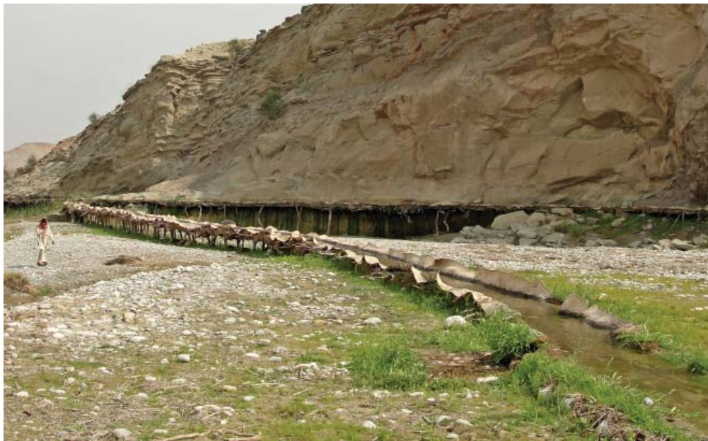
Figure 15. View of Madh, a traditional method of taking water to agricultural land in Khirthar, Sindh.
